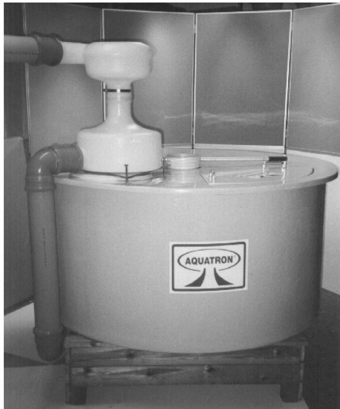
**Figure 5: Fluid outlet from Aq 4x300 system showing the 4" vertical connection pipe**
